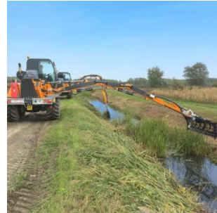
River Bucket for Vegetation Removal $8,917.89
