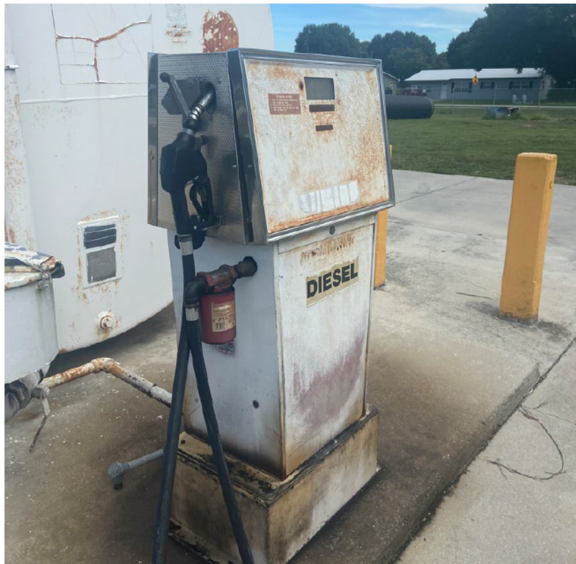
Existing Diesel Pump
