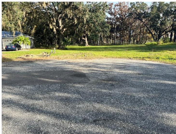
The Oaks Subdivision – Pavement depth thorough out the subdivision is minimal. We have had to perform frequent repairs to potholes and damage caused by trash trucks turning around at the end of the two cul-de-sacks.
